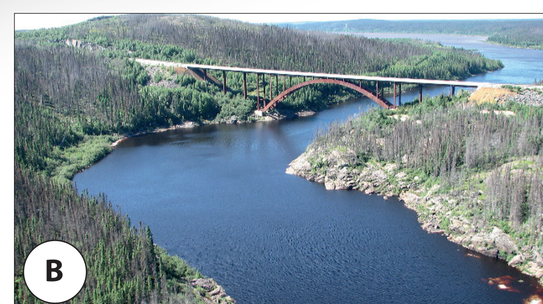
Eastmain River Bridge on the Highway
